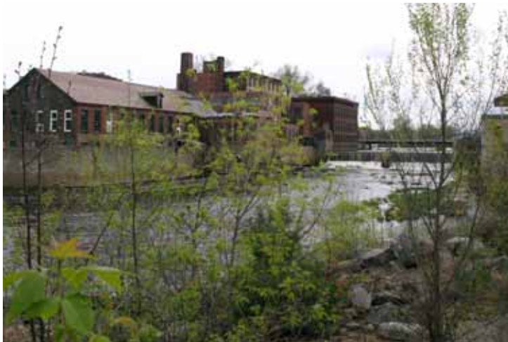
Former New Home Sewing Co. Buildings and dam in Orange.
