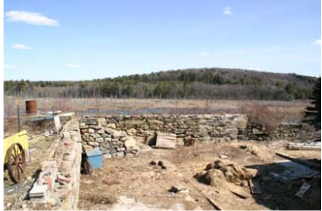
Silliman Barn foundation and Podunk Marsh in the distance
