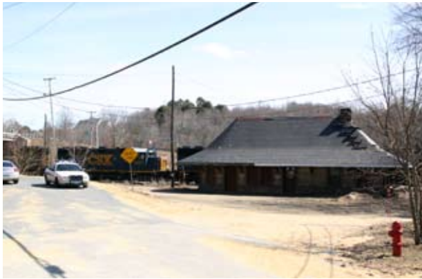
Freight trains still run behind the old station
